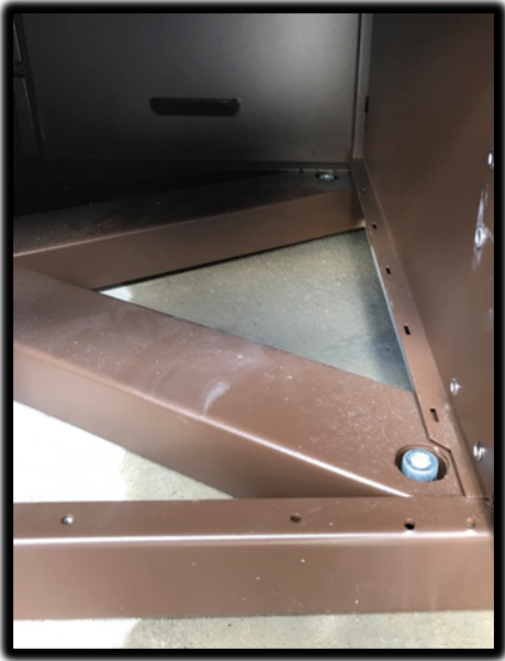
Leveling bolt hole locations under floor panels on corners of the frame.
